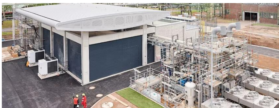
Figure 6: Hydrogen Fuel Generation System in Shell’s Energy and Chemicals Park Rheinland, Germany
